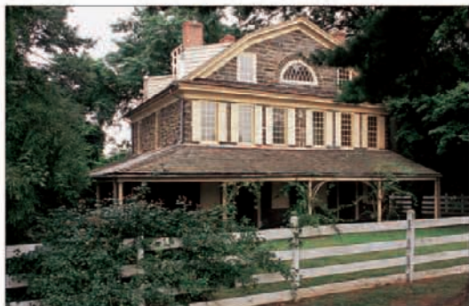
Cedar Grove, built as a summer home in 1750 ⑪
