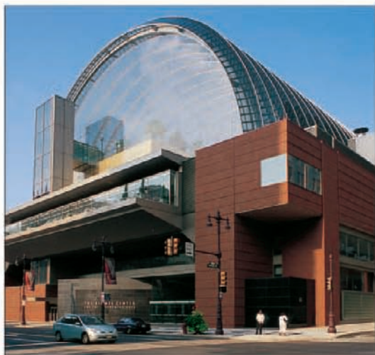
The Kimmel Center's glittering, modern façade
