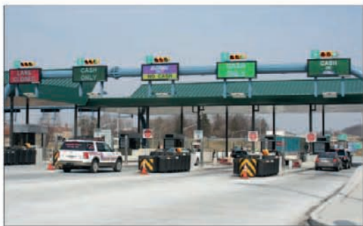
Toll booths on Interstate 76, Philadelphia
