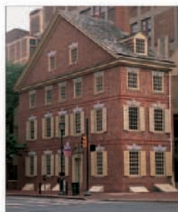
Declaration House, reconstructed in 1975 by National Park Service
