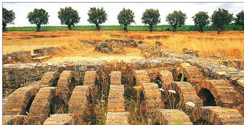
Remains of the hypocaust, the Roman underfloor heating system, at Vila Cardílio outside Torres Novas
