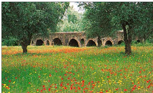
Roman bridge over the Odivelas, near Vidigueira
