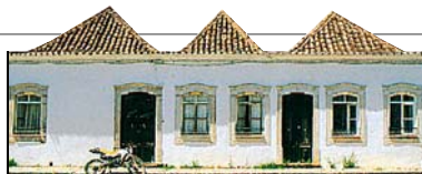
Telhados de quatro águas , the distinctive tiled roofs found in Tavira, the Algarve (see p332)
