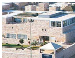
The modern complex of the Centro Cultural de Belém
