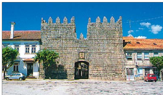
The main gateway into the old walled town of Trancoso
