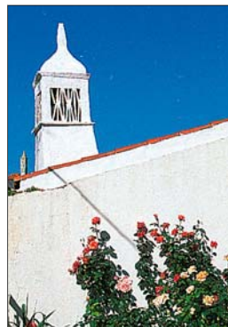
One of many filigree chimneys that adorn the rooftops of Alte
