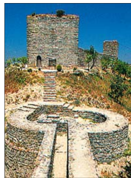
Ruined secret passage connecting the towers of the castle in Ourém
