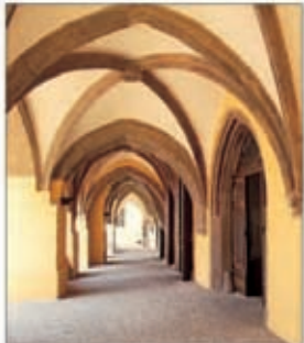
Týn School Gothic rib vaulting is a primary feature of this building, which was a school from the 14th to the mid-19th century.
