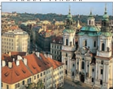
Aerial view of the Baroque Church of St Nicholas in the Old Town Square
