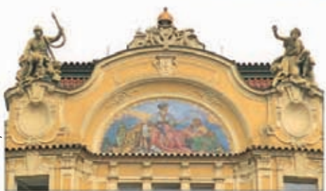
Ministerstvo pro místní rozvoj Architect Osvald Polívka designed this Art Nouveau building in 1898, with figures of firefighters on the upper façade. It houses the Ministry of Local Development.
