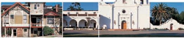
Left Victorian houses in Heritage Park Right Façade of Mission San Luis Rey de Francia
