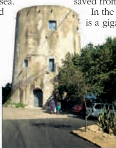
The Aragonese tower at Santa Maria Navarrese
