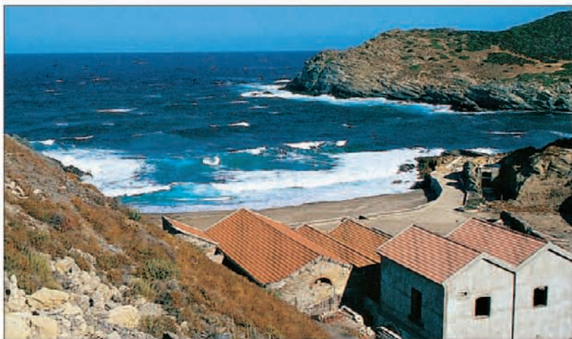
The old mine buildings at Argentiera
