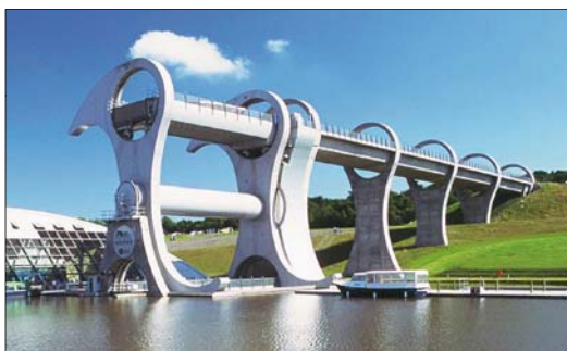
The rotating Falkirk Wheel boat lift
