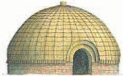
Zulu "beehives" are a community effort. The stick framework is erected by the men, and the women thatch it.
