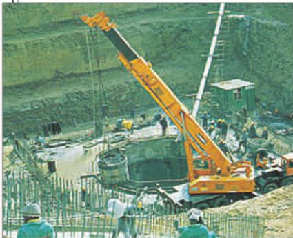
The main shaft , sunk to a depth of 60 m (197 ft), is encased in a concrete "collar" to support the headgear. South African gold-mine shafts are the deepest in the world, because the reefs are located several miles underground.
