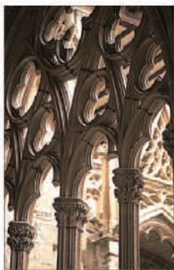
Stone tracery in the elegant cloister of Pamplona cathedral
