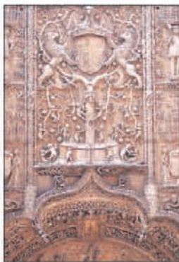
Façade of Colegio de San Gregorio, Valladolid
