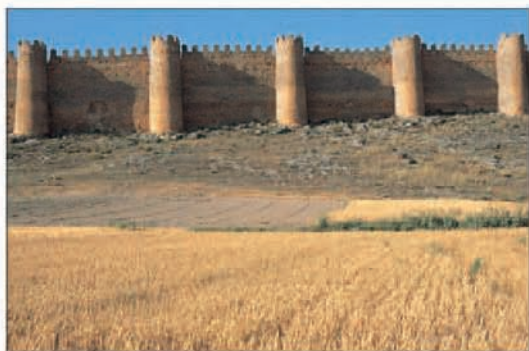
Curtain walls and drum towers of Berlanga de Duero castle
