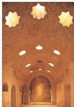
Horseshoe arches supporting the dome at the Baños Árabes, Jaén
