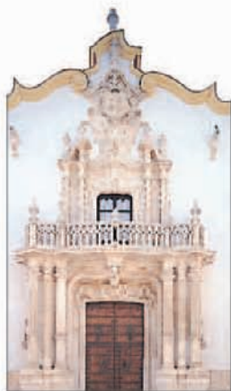
Palacio del Marqués de la Gomera, in Osuna, completed in 1770
