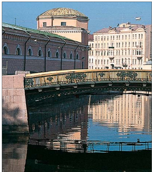
North façade of Imperial Stables (left) and Little Stable Bridge on the Moyka
