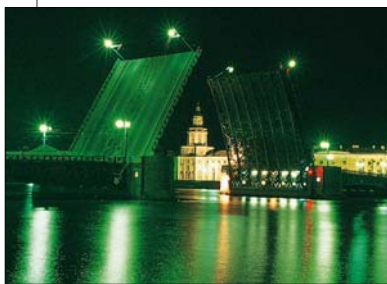
Dvortsovyy most (leading to Vasilevskiy Island), raised to allow ships access along the Neva
