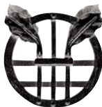
Kshesinskaya Mansion railing detail
