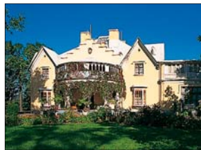
Cottage Palace in Alexandria Park
