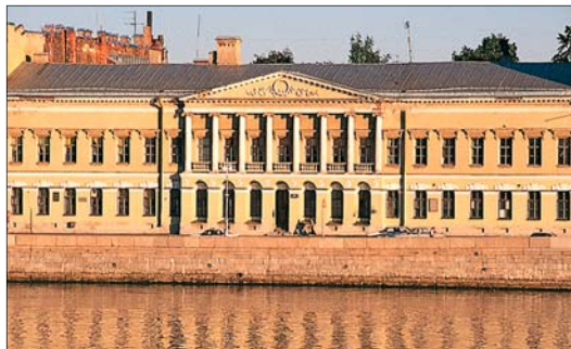
Quarenghi's grand porticoed façade, at No. 32 on the English Quay
