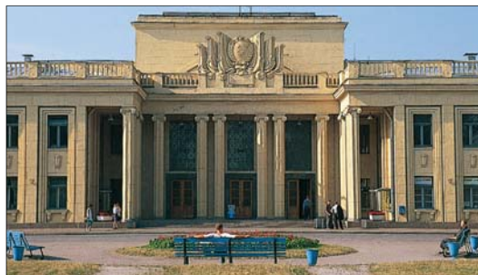
Stalinist architecture at Pulkovo 2, St Petersburg's international airport
