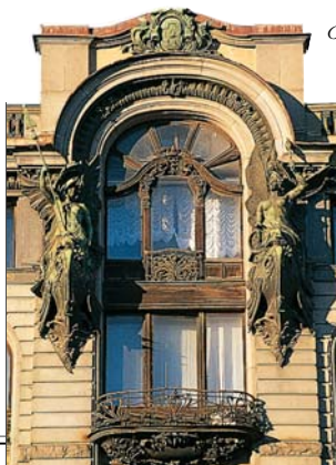
Singer House (1910–14) reveals Pavel Syuzor's use of an unusually eclectic mix of architectural styles. Ornate Style-Moderne wrought-iron balconies and decorative wooden window frames combine with elements of Renaissance and Baroque revivals.
