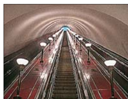
Step escalators to platforms
