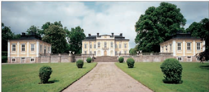
Steninge Palace, one of the most perfect examples of late 17th-century manor house design
