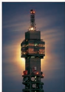
Kaknästornet, Stockholm's tallest building at 155 m (508 ft)
