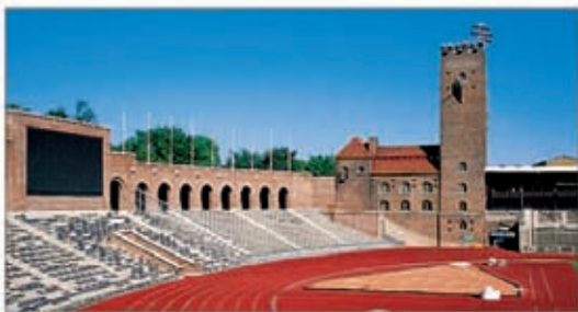
Running track at Stadion, 1912
