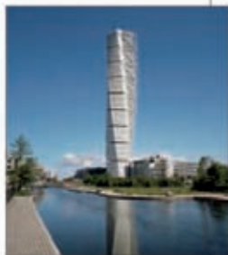
The Turning Torso building soaring 190 m (623 ft) high
