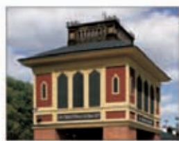
Hauling plant at the Sala silver mine, in use until 1908
