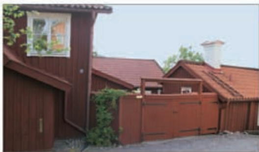
Red-painted, 18th-century wooden buildings in central Strängnäs
