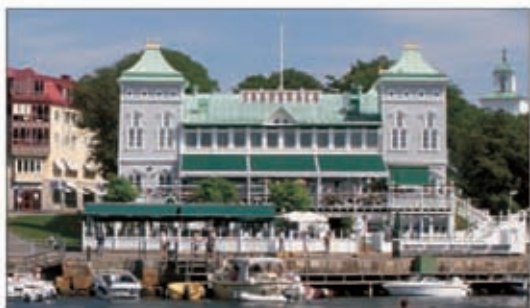
Hotell Skagerack on the harbourfront in Strömstad
