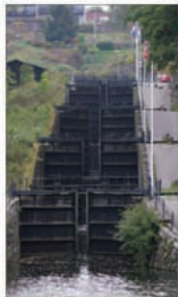
Staircase of locks on the Trollhättan Canal, rising 32 m (105 ft)
