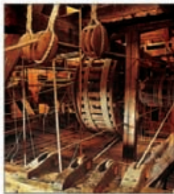
Court Theatre stage machinery dating from 1766
