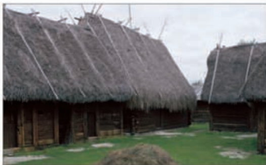
Buildings at Bungemuseet with thatched roofs of Gotland sedge
