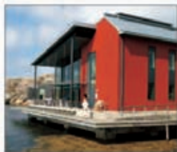
The Watercolour Museum, Tjörn, resting on piles in the water
