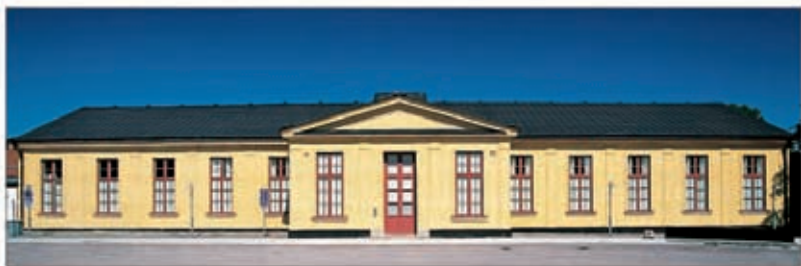
Arkitekturmuseet, housed in the Neo-Classical former naval drill hall
