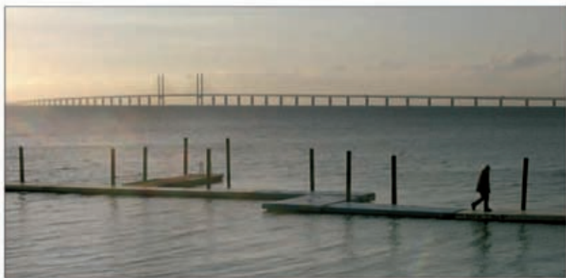
The 8-km (5-mile) long Öresund Bridge between Sweden and Denmark, carrying a motorway and railway line
