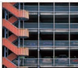
Multistorey car park in Geneva
