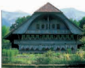
Rural house typical of the Bern region of the Mittelland during the Baroque period. The roof is designed to enable it to withstand heavy coverings of snow.
