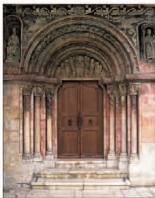
Portal of the church at St-Ursanne
