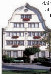
House in Gais, with an ornate gable
