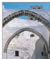
Arched buttresses for earthquake protection
