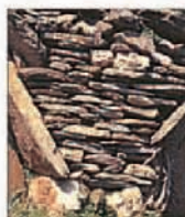
Unmortared wall of schist slabs
