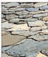
Slate (or "fish-scale") roof
