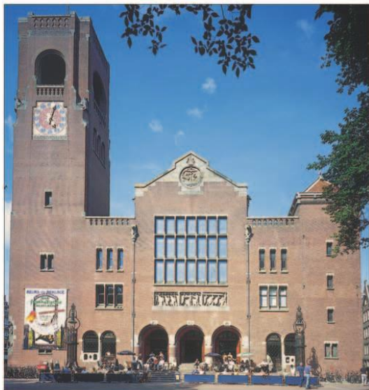
Decorative brickwork on the façade of the Beurs van Berlage
