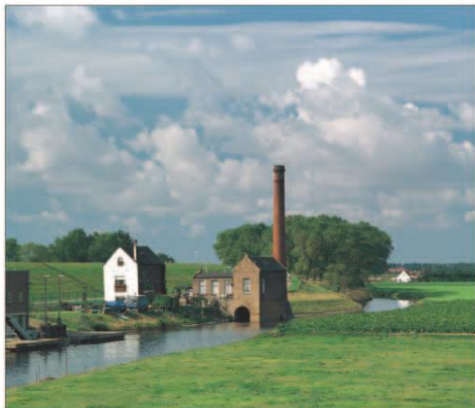
Pumping station in a rural setting in the neighbourhood of Tholen
