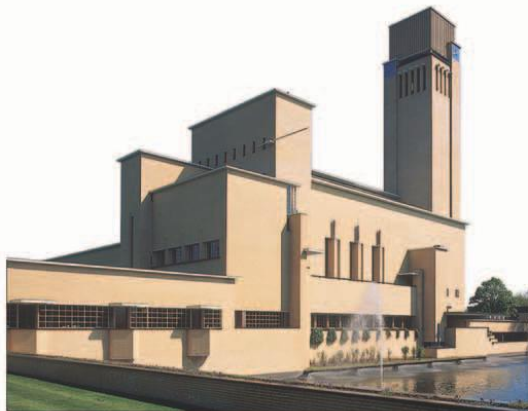
Hilversum town hall, finished in yellow brick
