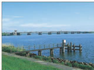
The Ketelbrug bridge over the Ketelmeer
