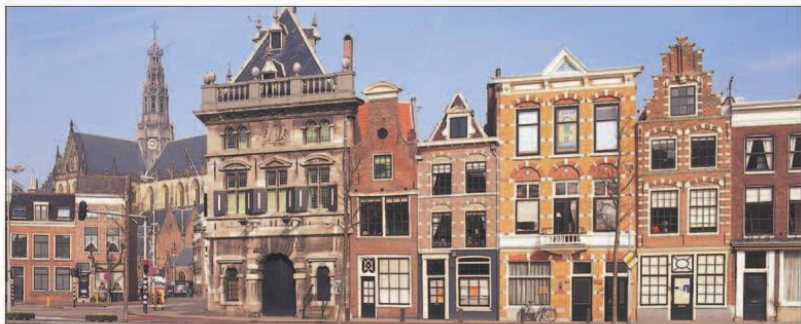
17th- and 18th-century gabled houses along the river Spaarne in Haarlem
