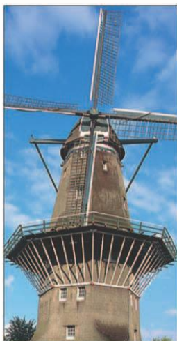
The 18th-century De Gooyer windmill, with its renovated balcony
