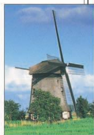
Watermill in the Schermer polder
