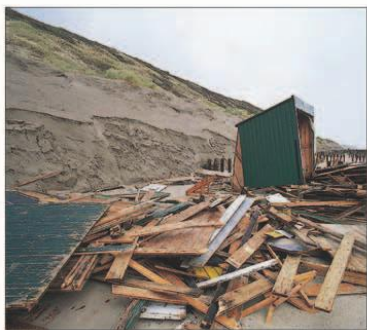
The Dutch coast seriously damaged by storms
