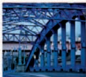
Komagata Bridge over Sumida River
