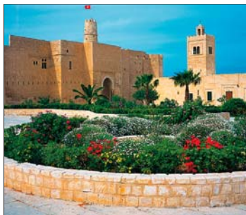
Great Mosque, standing next to the ribat
