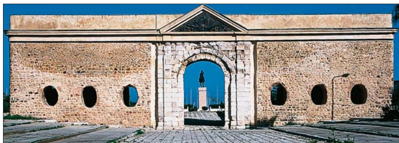
Remains of an 18th-century arsenal, constructed by Hammouda ibn Ali Bey, in La Goulette
