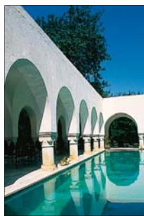
Villa in Hammamet, an early 20th-century Modernist house owned by George Sebastian.
