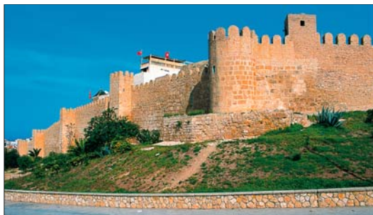
Walls of the medina, dating from the 9th century
