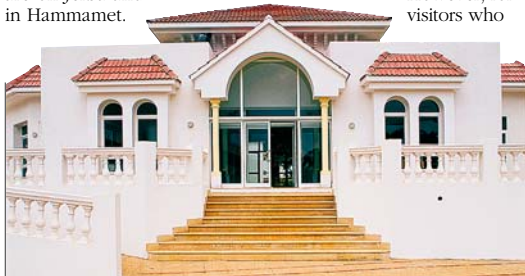
The main pavilion of the Hammam Bourguiba resort
