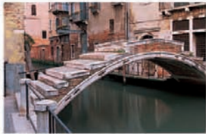
Bridge with No Parapet
