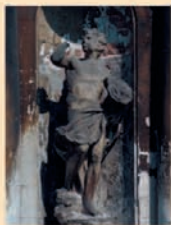
Stonework damaged by waves
