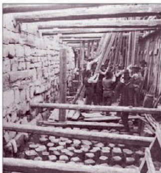
Strengthening the Campanile foundations
