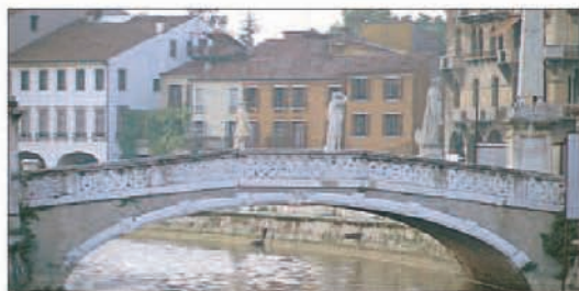
One of four stone bridges spanning the canal around Prato della Valle
