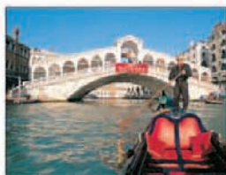
The Rialto Bridge, on the Grand Canal
