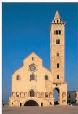
The facade of Trani's Duomo
