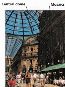
Galleria Vittorio Emanuele II in Milan, designed by Mengoni in 1865, was the first Italian building to use glass and iron structurally (see p194).
