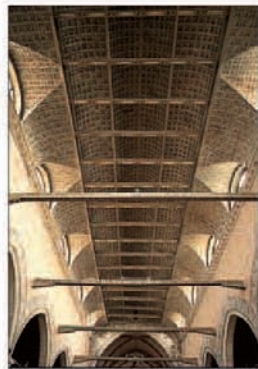
The ceiling of Santo Stefano, built in the form of a ship's keel
