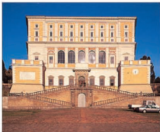
The main facade of the pentagonal Palazzo Farnese at Caprarola
