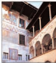
Inner courtyard of the Magno Palazzo
