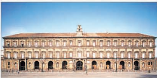
The facade of the Palazzo Reale, Naples' royal palace
