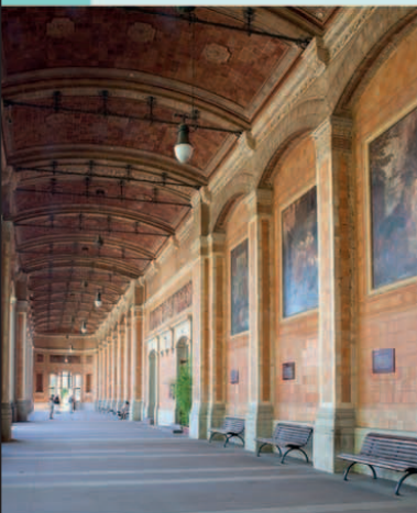
Above Interior of the grand Trinkhalle, Baden-Baden
