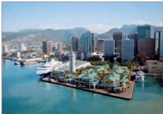
View of Aloha Tower Marketplace and the Honolulu Harbor
