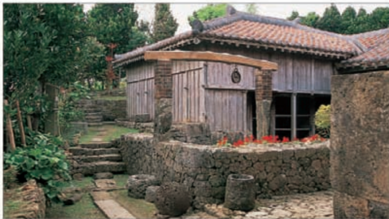
Part of the Nakamura House on Okinawa, a fine example of traditional architecture
