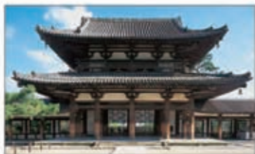
Gate at the Horyu-ji compound
