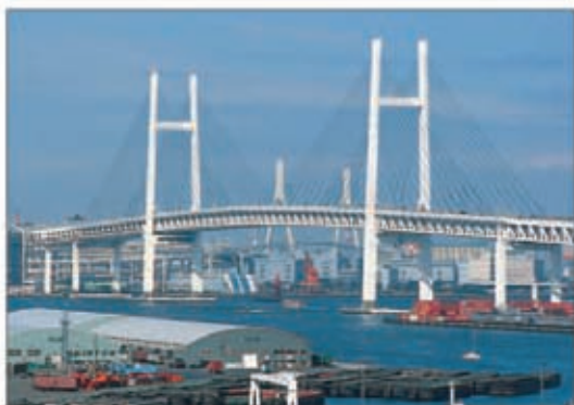
Yokohama Bay Bridge
