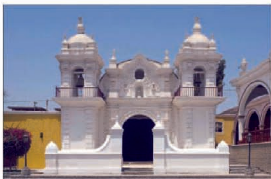
Chapel façade at Hacienda San José prior to earthquake damage
