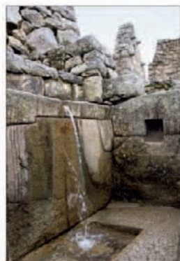
Water collects in the cut stone base of the fountains
