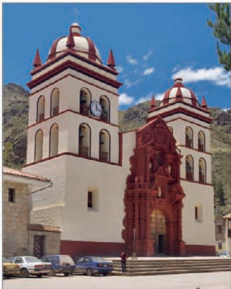
Brightly-colored façade of the Cathedral in Huancavelica, one of the best examples of Colonial architecture in the region
