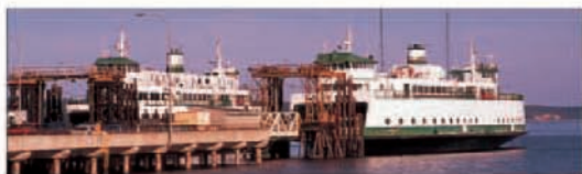
Washington State Ferries terminal, Port Townsend
