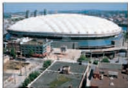
The enormous air-supported dome of BC Place Stadium
