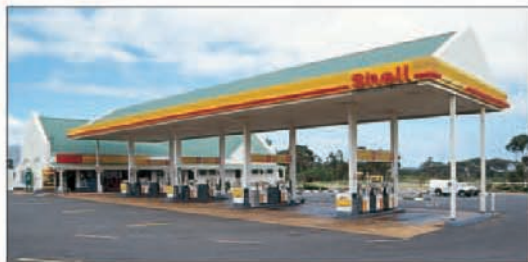
A gas station, one of many on major highways and in towns and cities
