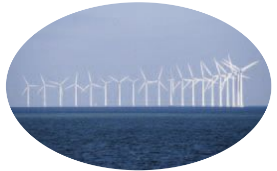
Offshore wind farm
