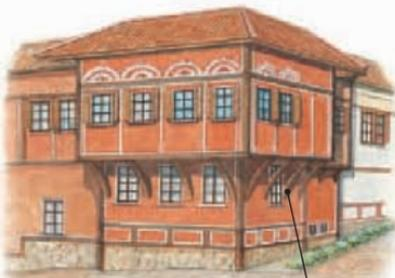
Cantilevered upper storey makes best use of limited ground space.
