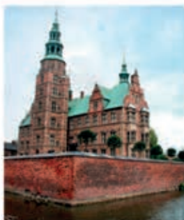
MOAT A wide, steep-walled ditch around the castle, usually filled with water.
