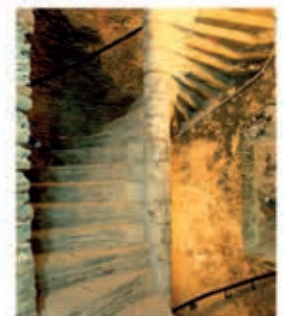
SPIRAL STAIRCASE Narrow, spiral staircases meant that invaders could not easily use swords while climbing.
