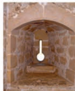
ARROW AND GUN LOOPS The thick walls had narrow slits through which a soldier could fire missiles at attackers.
