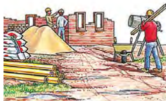
A construction site .
