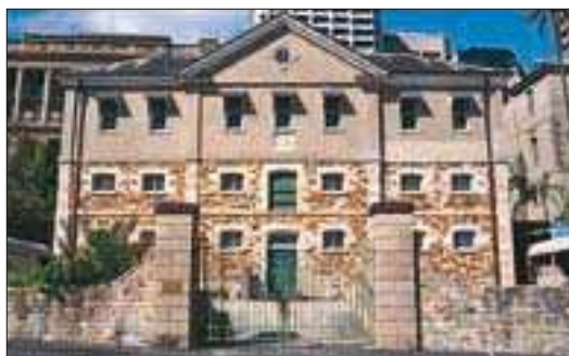
South façade of the restored colonial Commissariat Store Museum
