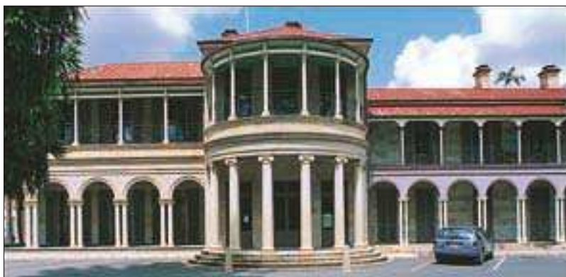
Arcade and arches of the north façade of Old Government House
