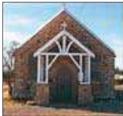
Simple façade of the Holy Trinity Church in Roebourne
