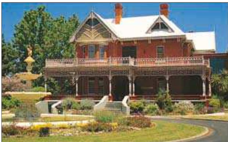
Rio Vista, the elaborate home of irrigation expert William Chaffey, in Mildura
