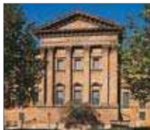
Museum Entrance The façade features massive Corinthian square pillars or piers.
