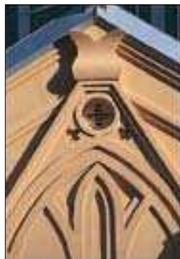
Roof detail of St Francis' Church
