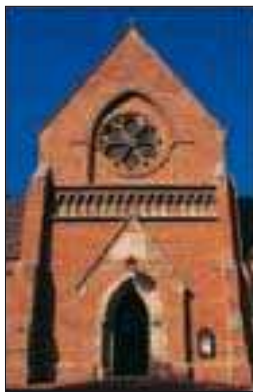
Western façade of St George's Cathedral showing rose window
