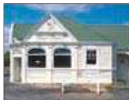
Typical 19th-century building in Bothwell
