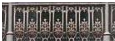
Cast-iron lacework at Tasma Terrace
