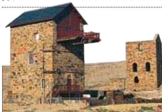
Restored 19th-century buildings at Burra Mine near the Clare Valley
