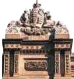
Detail of the ornate front parapet of Edmund Wright House
