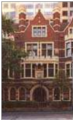
Chambers at No. 120 Collins Street
