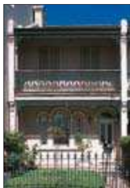
Paddington Street terrace house
