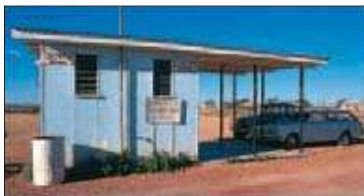
Tiny domestic terminal in Birdsville, Queensland
