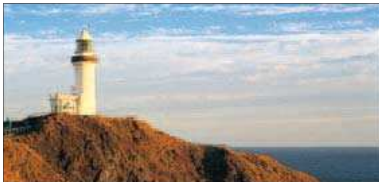
Cape Byron lighthouse on Australia's most easterly point
