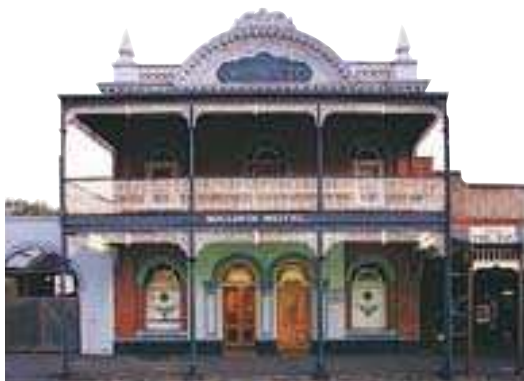
Typical 19th-century building in Maldon
