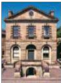
The former Governor's house, Old Gaol, Darlinghurst
