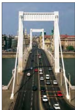
1964 The Elizabeth Bridge (see p63) reopens to traffic, having been totally reconstructed
