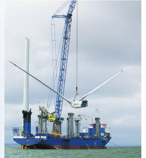
Most wind turbines resemble aircraft propellers
