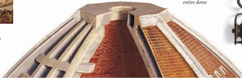
The weight of the lantern helps to stabilize the structure of the entire dome
