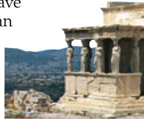
THE ERECHTHEION A smaller temple than the Parthenon, the Erechtheion, called after a legendary king of Athens, probably housed the wooden statue of Athena. Its famous porch has marble statues of women ( caryatids ) instead of columns, holding up the roof.
