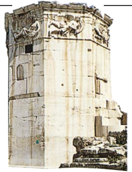
TOWER OF THE WINDS In the 1st century B.C., the Greek astronomer Andronicus built a horologium, or tower of winds. The tower was octagonal (eight-sided), and on each face was carved one of the eight wind spirits, one for each direction the wind blew. Boreas (north wind) and Notos (south wind) were the main winds.
