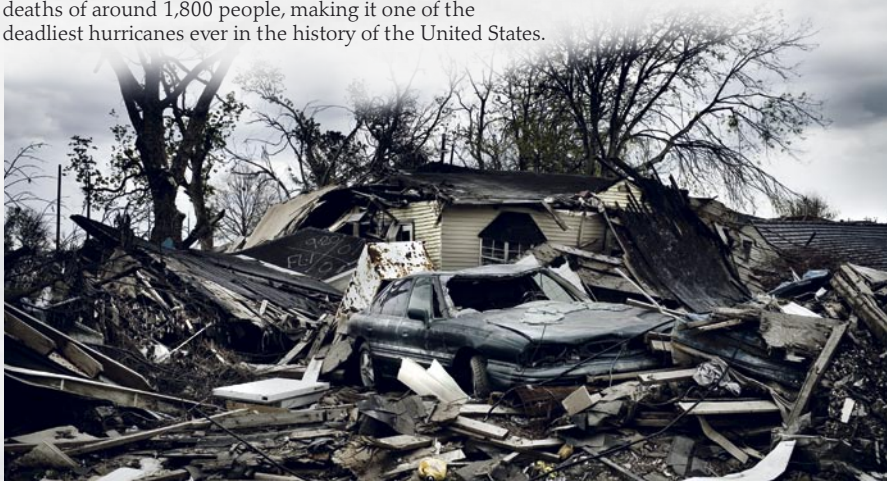
Damage from Hurricane Katrina
