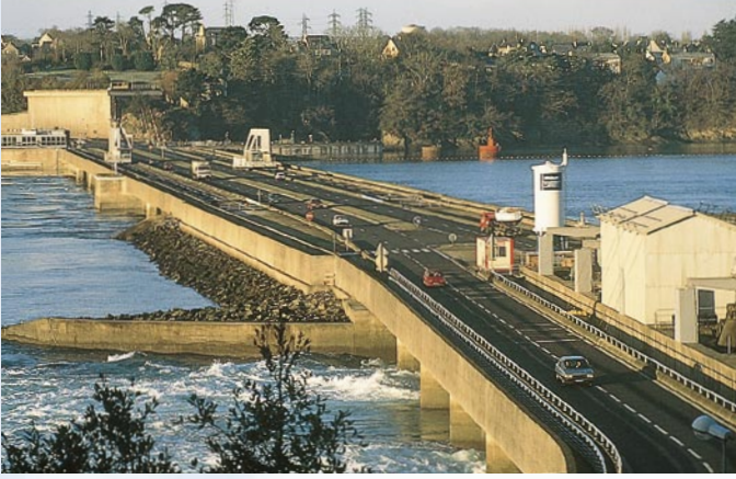
La Rance tidal barrage, France
