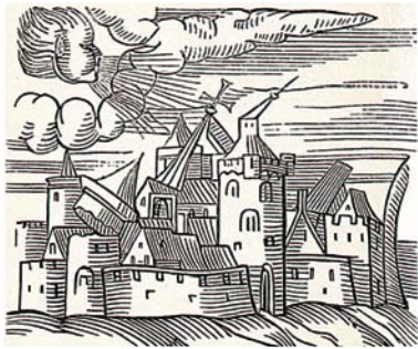
Hurricane force winds often damage buildings
