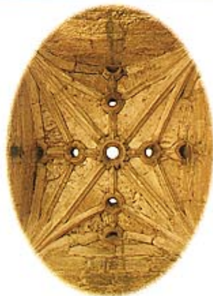
DROPPING IN The gate passage at Bodiam has so-called "murder holes" ( meurtrières ) in the roof so cold water could be poured down to put out fires. Scalding water, hot sand, or other offensive substances might be also dropped on enemies who managed to get in.
