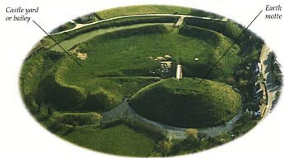
PLESHEY The large motte and bailey at Pleshey, England, was built by the Normans soon after 1066. This type of castle could be erected in a matter of months rather than years, which was ideal when the Normans were in a hostile country. Pleshey castle has one motte and one bailey, but sometimes there were two mottes or two baileys.
