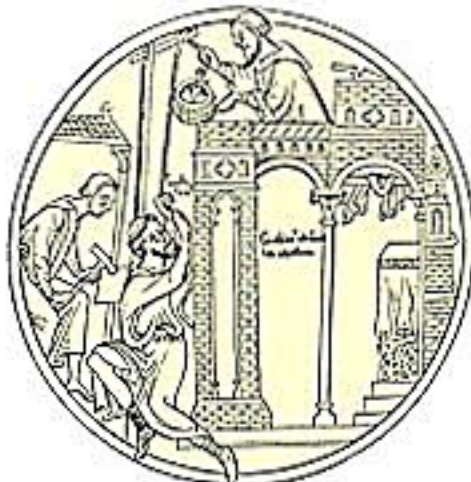
STONE ME A 13th-century mason wearing a cloth coif on his head shapes stone blocks while a basket of stone is sent up to the workman waiting at the top of the building.
