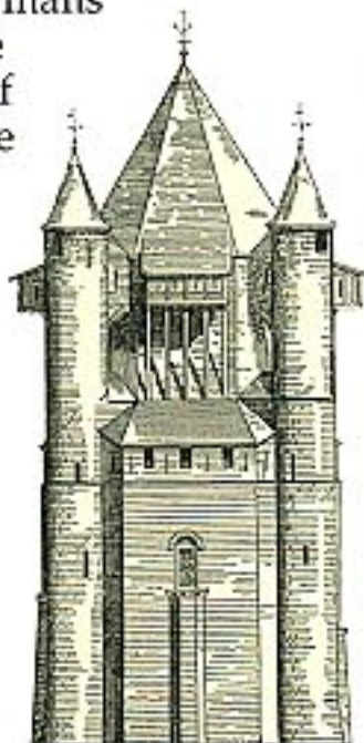
HOARDINGS The octagonal tower at Provins, France (built in about 1150) is shown here with wooden hoardings (pp. 28–29) that were added later.
