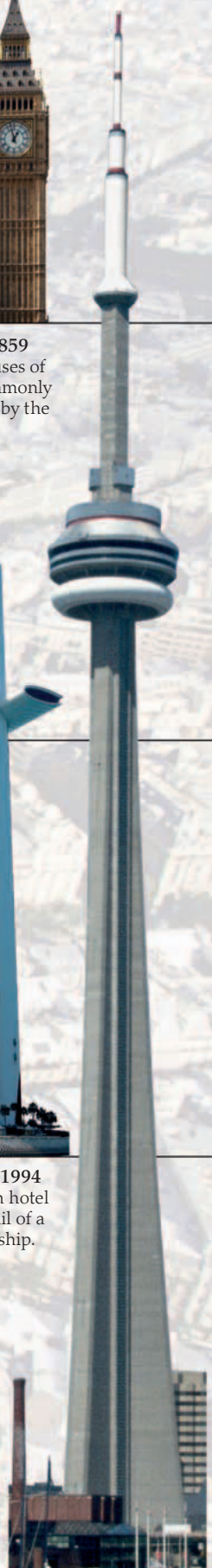
CN TOWER, TORONTO, 1973-76 This broadcasting tower was the tallest in the world until 2007, when Burj Khalifa, Dubai, surpassed it.
