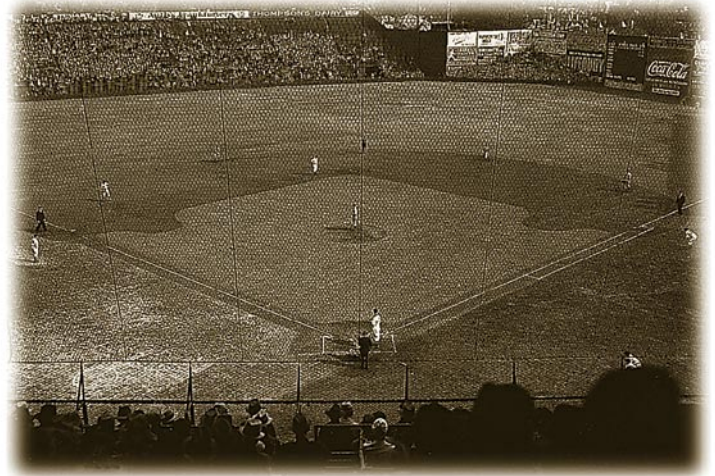
DIAMONDS OF OLD This photo of Griffith Stadium from 1933 shows that diamonds haven't changed much from earlier times. A wide dirt area separated the infield grass from the outfield grass. This view also shows the netting that ballparks put up behind home plate to protect fans from fast-moving foul balls or wild pitches.
