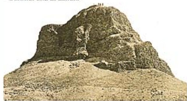
THE BLACK PYRAMID Senusret III and his successor Amenemhat III built their pyramids at Dahshur, just south of Saqqara. This is Amenemhat III's pyramid, often called the Black Pyramid. Like most Middle Kingdom pyramids, it is now just a pile of rubble. The core of mud bricks has subsided over the centuries, and the fine stone facings were plundered for later building projects. The corridors and chambers, including the tombs of at least three queens, were dug about 12 m (40 ft) underground. But the king's burial chamber with its beautiful granite sarcophagus was never used.
