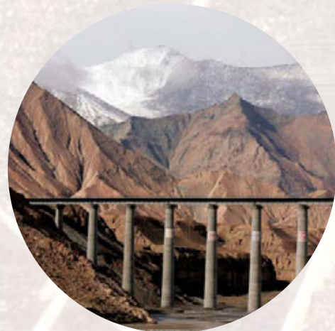
● QINGZANG RAILROAD (CHINA) This 1,215-mile (1,956-km) route from Lhasa, Tibet, to Xining, Qinghai Province, includes the world's highest section of track through the Tanggula Pass at 16,640 ft (5,072 m). To make travel at high altitude easier, the cars have an oxygen supply for each passenger.
