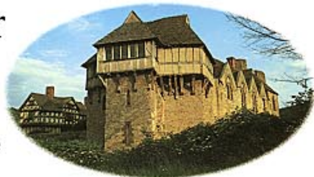
HOME DEFENCE Stokesay is a fortified manor house in Shropshire, England. It consists of a hall and chamber block with a tower at each end, mostly built in the late 13th century. In the 17th century a half-timbered gallery was added.
