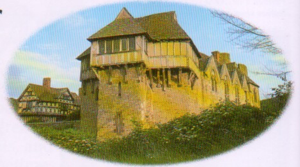
HOME DEFENCE Stokesay is a fortified manor house in Shropshire, England. It consists of a hall and chamber block with a tower at each end, mostly built in the late 13th century. In the 17th century a half-timbered gallery was added.
