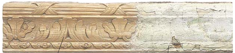
Wood stripped clean to show original carving
