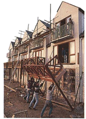
HEAVE HO! A wooden balcony and its supports are often made separately before being attached to the wall of a building. Once this balcony has been pushed into position and fixed, most of its weight will be carried by the wooden uprights.
