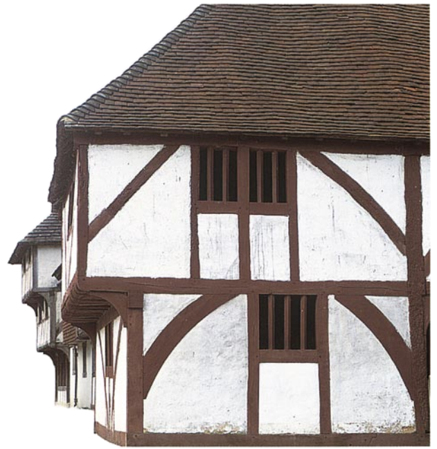
Jettied timber-framed houses, England
