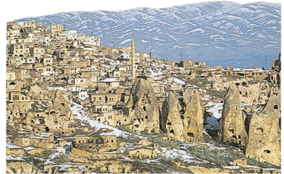
HANGING HOUSES Houses were sometimes built on rocky outcrops for defensive purposes. After the Middle Ages, with the introduction of gunpowder and the change in the ways wars were fought, defense of individual buildings became less important. Houses were given larger windows, and even ornate wooden balconies like these at Cuenca in Spain.
