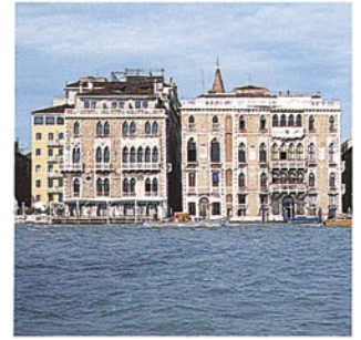
CITY ON THE WATER Venice is built on islands in a lagoon. The buildings are supported on massive piles of pinewood that were sunk deep into the sand and clay beneath the water. Foundations of Istrian limestone resist corrosion from the seawater. The houses are connected by a network of narrow streets and by some 100 canals crossed by more than 400 bridges.
