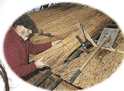
Steel sway holds reeds in place
