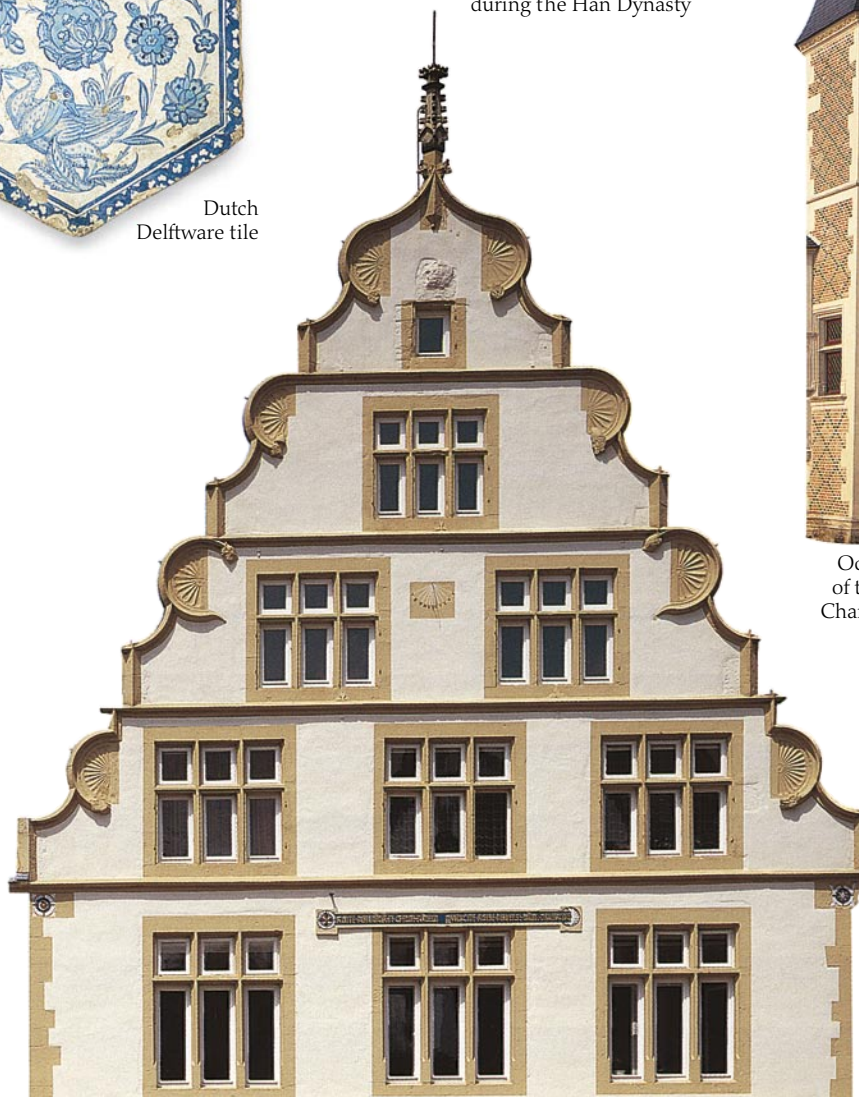
Gabled town house, Lemgo, Germany
