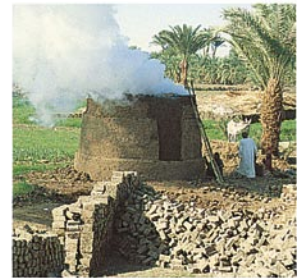
Firing bricks in a kiln at Luxor in Egypt
