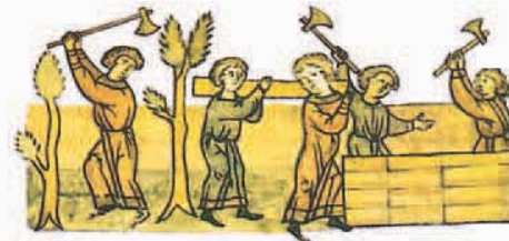
THE WALLS GO UP
