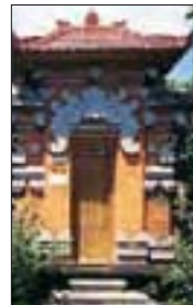
Gate with decorated roof and brickwork
