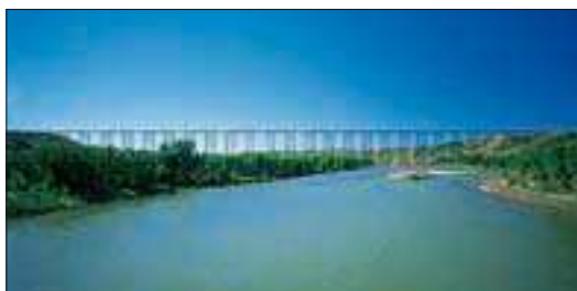
Iron Bridge over the Oldman River, Lethbridge
