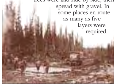
Bogged-down truck waits for corduroy to be laid
