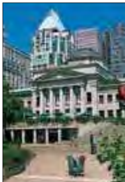
Decorative Victorian features on the Vancouver Art Gallery façade
