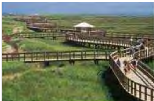
The raised boardwalk at the Irving Eco-Centre, La Dune de Bouctouche
