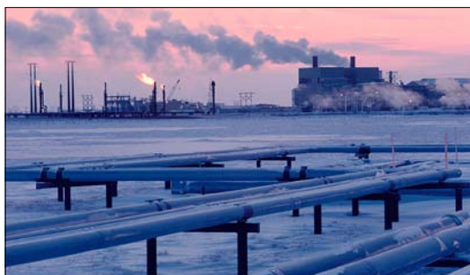
Pipelines crisscrossing the oilfields at Prudhoe Bay on the North Slope
