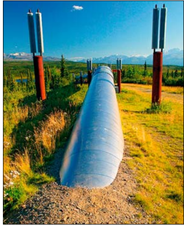
Alaska Pipeline with the backdrop of the Alaska Range
