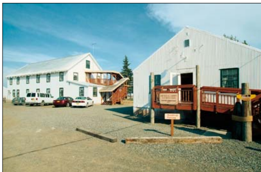
The old salmon cannery complex at Kenai Landing, Kenai
