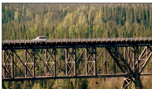
The narrow Kuskulana Bridge 283 ft (85 m) above the Kuskulana River
