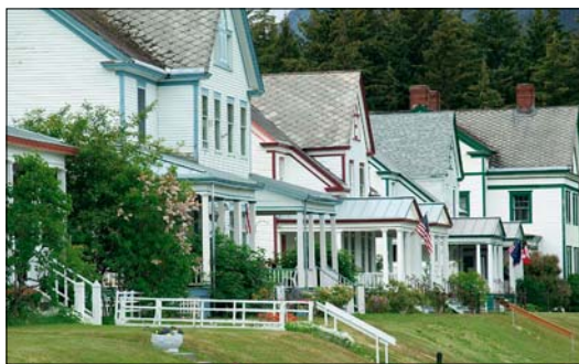
Former officers' quarters at Fort Seward, Haines
