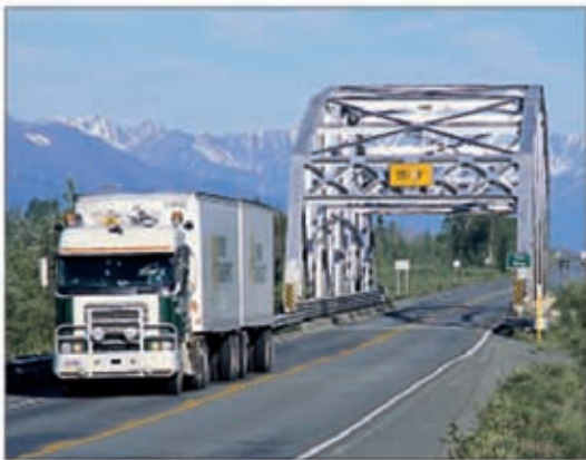
Truck hauling freight over Tok River Bridge east of Tok
