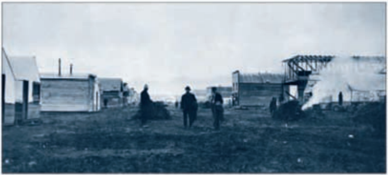
Timber structures being built on Main Street in Anchorage in 1915
