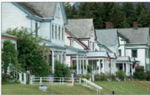
Former officers' quarters at Fort Seward, Haines
