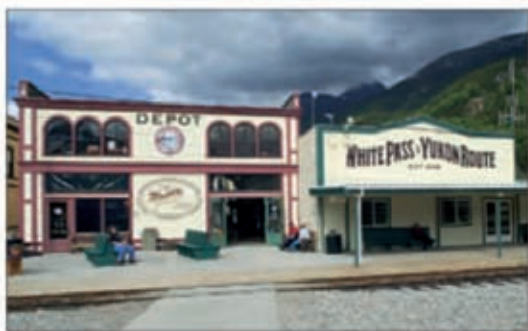
White Pass and Yukon Route Railroad depot, Skagway
