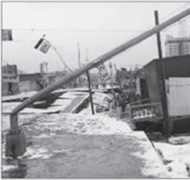
Anchorage's 4th Avenue a day after the massive 1964 Good Friday earthquake
