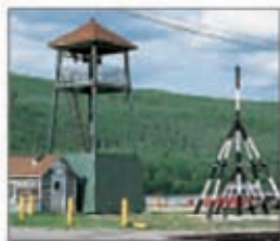
Four-legged "tripod" for determining ice breakup
