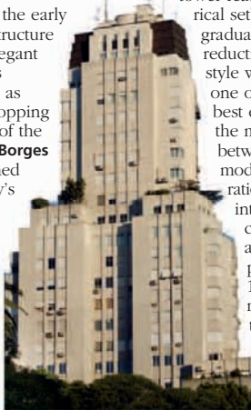
A view of the monolithic Edificio Kavanagh from Plaza San Martín
