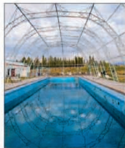
A thermal bath under an open sky in Pismanta
