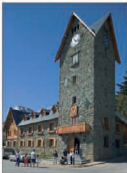
Municipal building and clocktower in Centro Cívico, Bariloche
