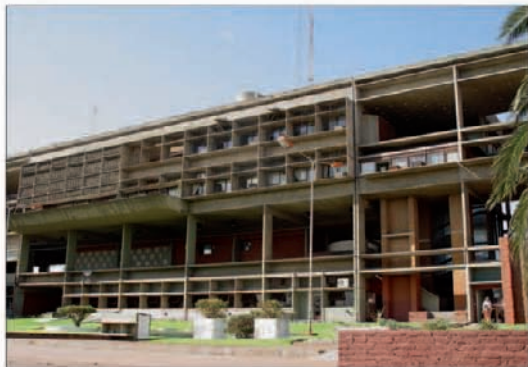
The Centro Cívico building at Santa Rosa
