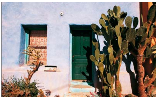
One of many 19th-century adobe houses in the Barrio Historic District
