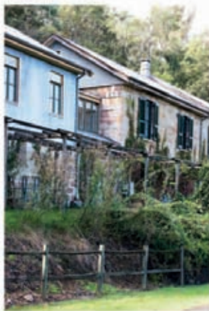
Above Buildings of the Tizzana Winery, Ebenezer
